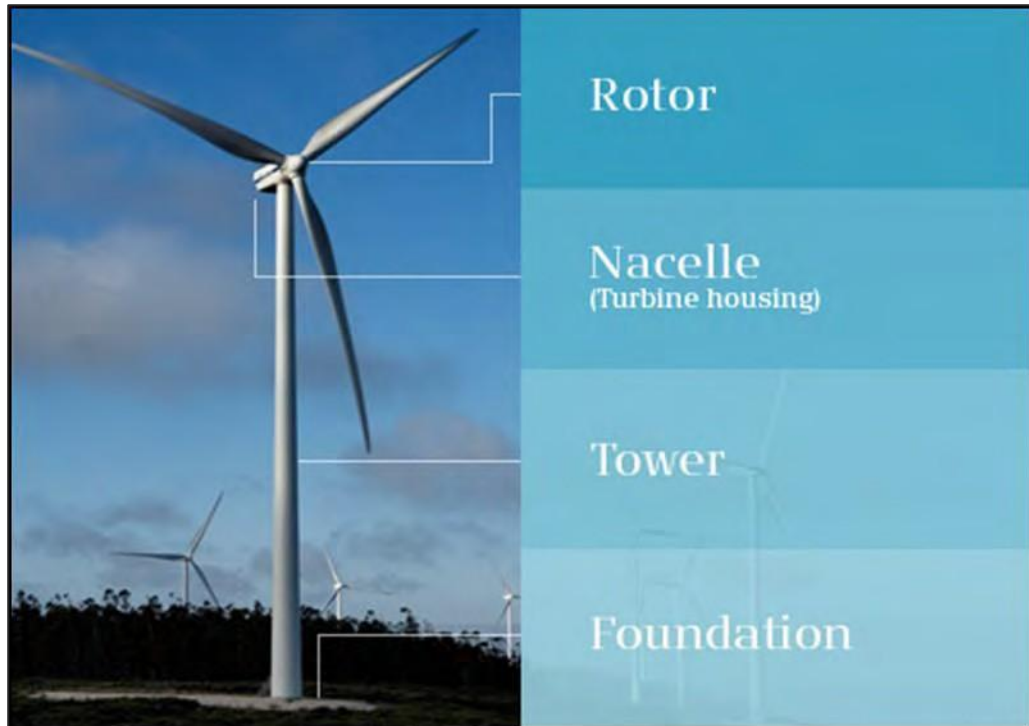
Figure 5-5: Typical Wind Turbine Components
