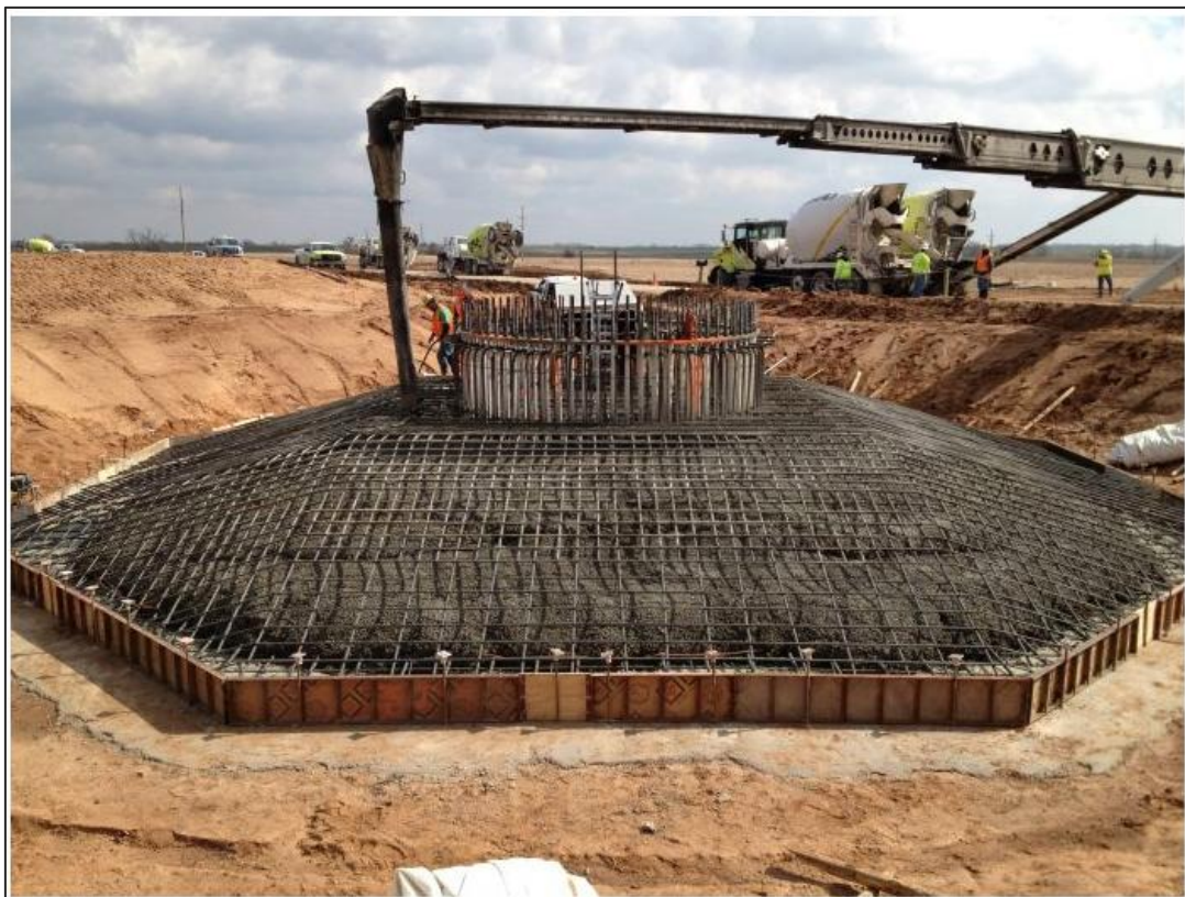
Figure 5-6: Typical Construction of a Wind Turbine Base (Source: www.windsystemsmag.com )
